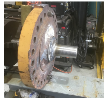
Condition of end cap and trunnion mount after pre-weld machining
